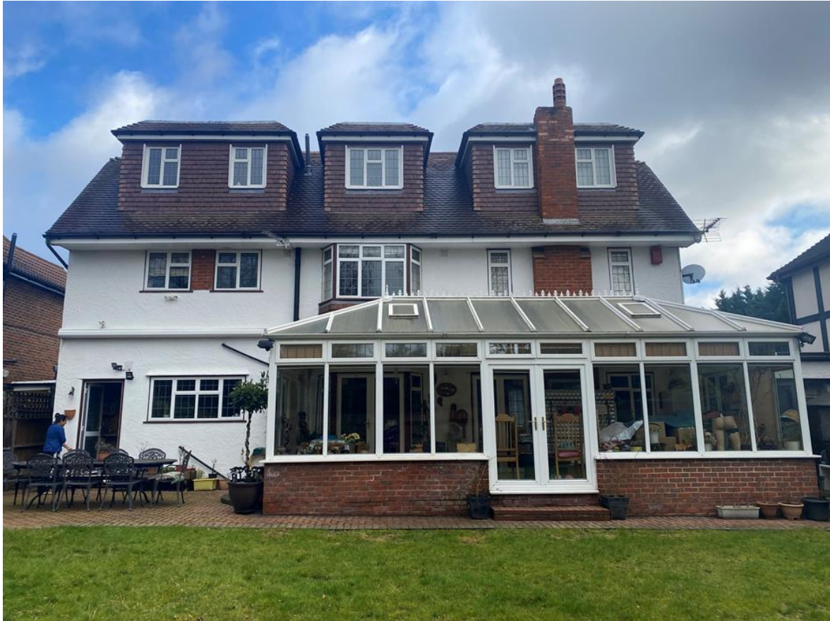
Figure 7: Photo of rear elevation
