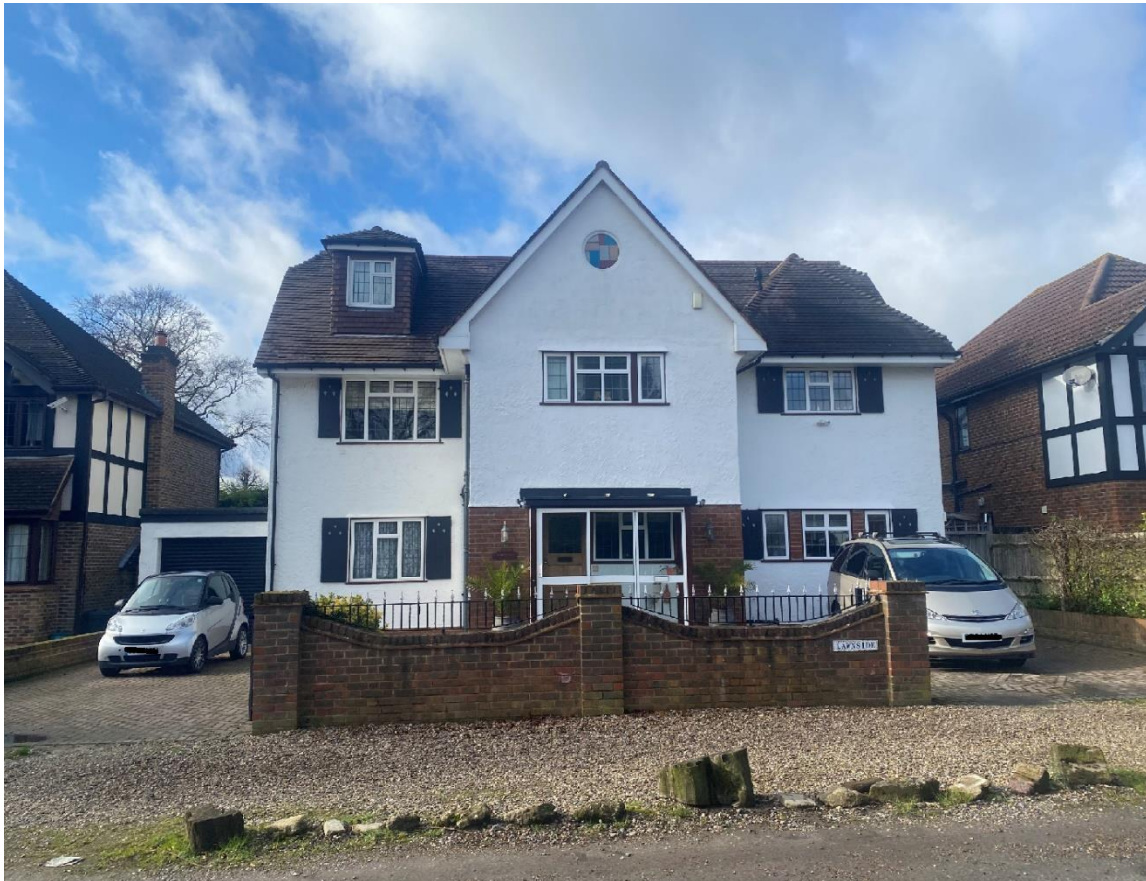
Figure 6: Photo of front elevation
